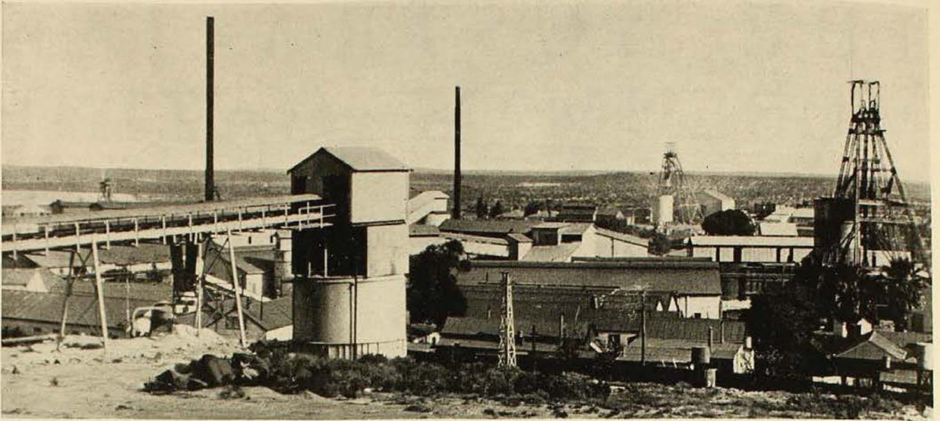
The southern end of Kalgoorlie's "Golden Mile." The ore bin in the foreground and the headframe in the distance belong to the Lake View and Star Group's Associated and Ivanhoe mines, respectively. On the extreme right is the headframe of the Perseverance mine, owned by Gold Mines of Kalgoorlie Ltd. The chimney stacks and buildings adjacent to them are the Kalgurli Ore Treatment Co.'s.
